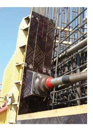
structure. Sheath thickness is chosen depending on the lateral pressure exerted in the curved sections and the movement of the strands during tensioning.
