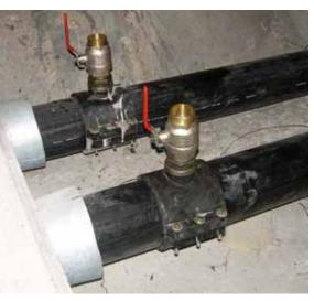
Injection inlets on HDPE pipes
