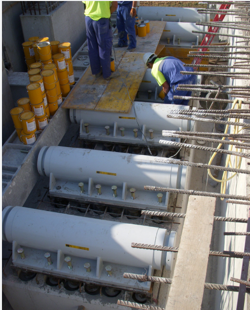
Longitudinal protection of a railway deck 8 units PDS 2200-3600-50
