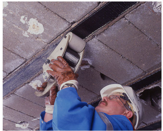
Application of the carbon fabric
